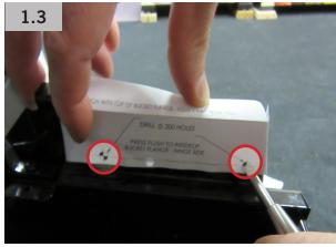
2.1 Using 3/16" drill bit, drill two holes on drop sensor mounting bracket in two locations from marks in Step 1.3 (**FIG. 2.1**).
