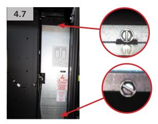
**NOTE:** Ensure that cover is not pinching wires.
