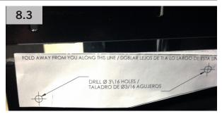
8.4 Using a spring punch or other marking device, place mark through template and onto bracket in two places where holes will be drilled in Step 8.5 (**FIG. 8.4**).
